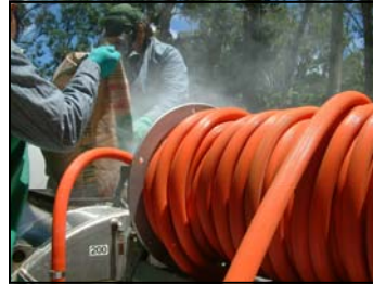
Crew mixing lime in sprayer
